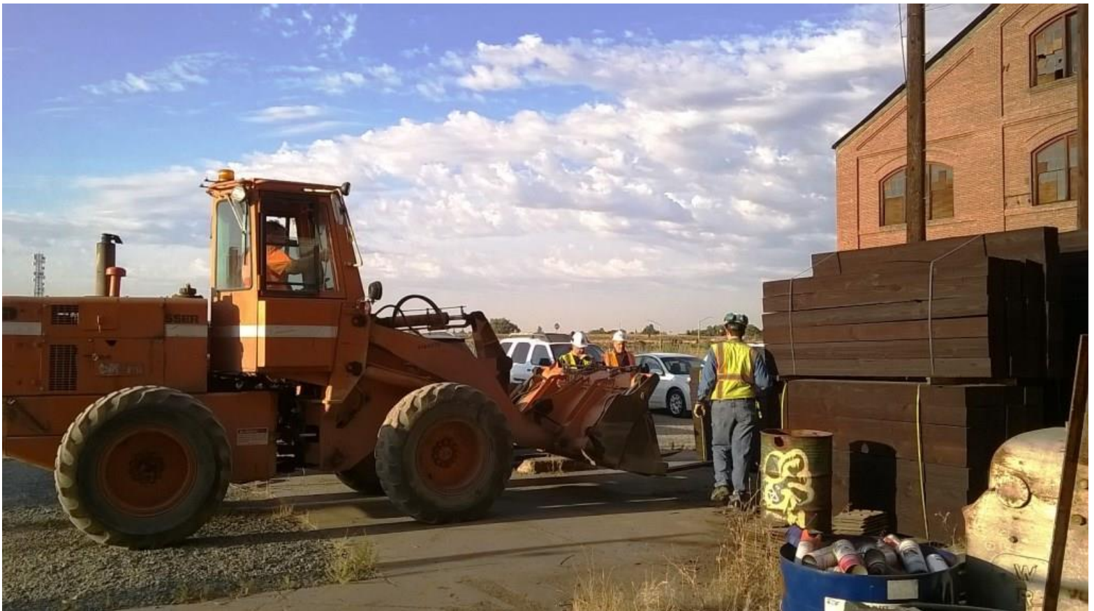
Frank in the loader grabs a bundle of ties
