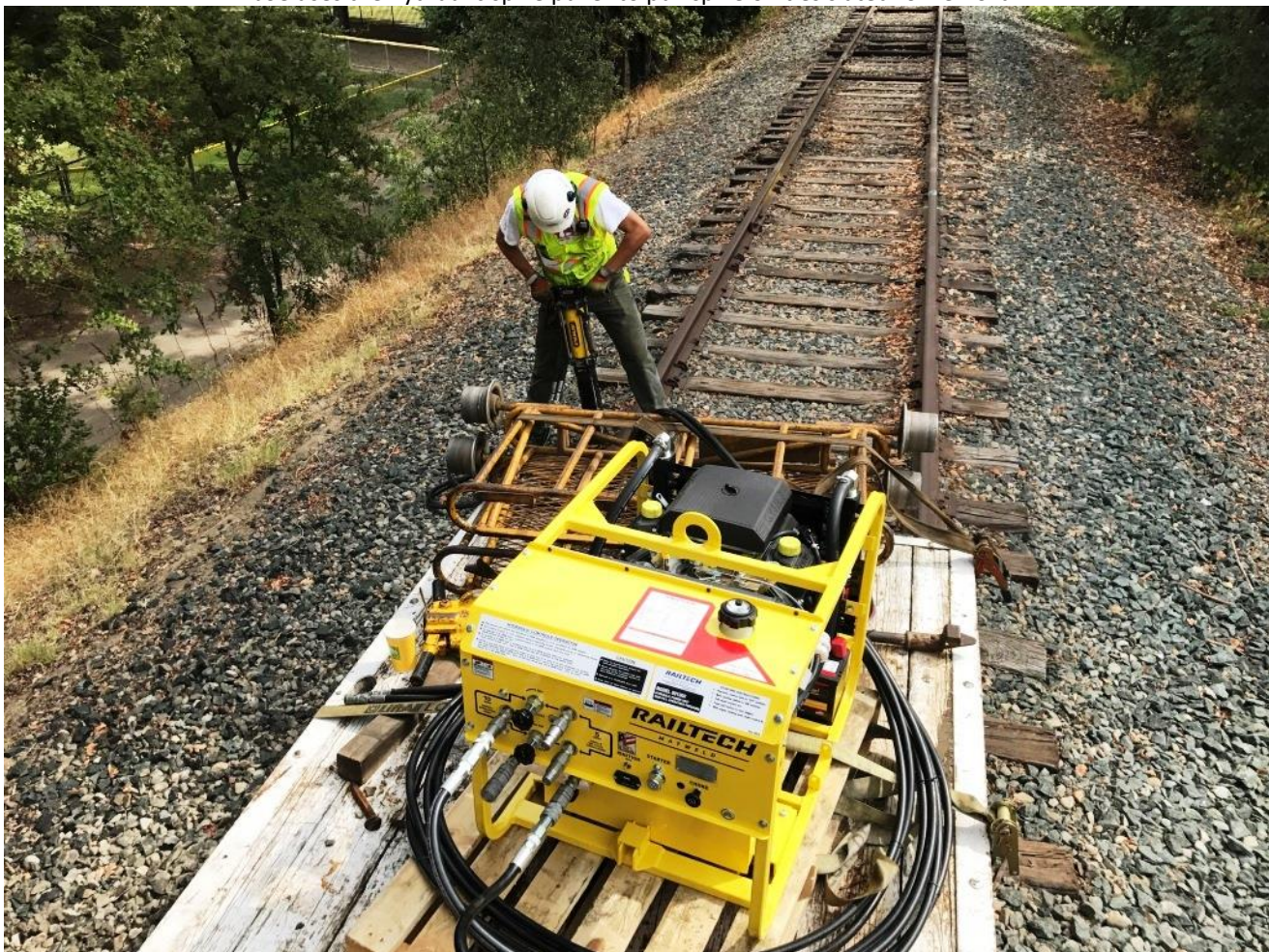
Kyle demonstrates how our super-duper new hydraulic power unit makes the hard job of pulling spikes super easy
