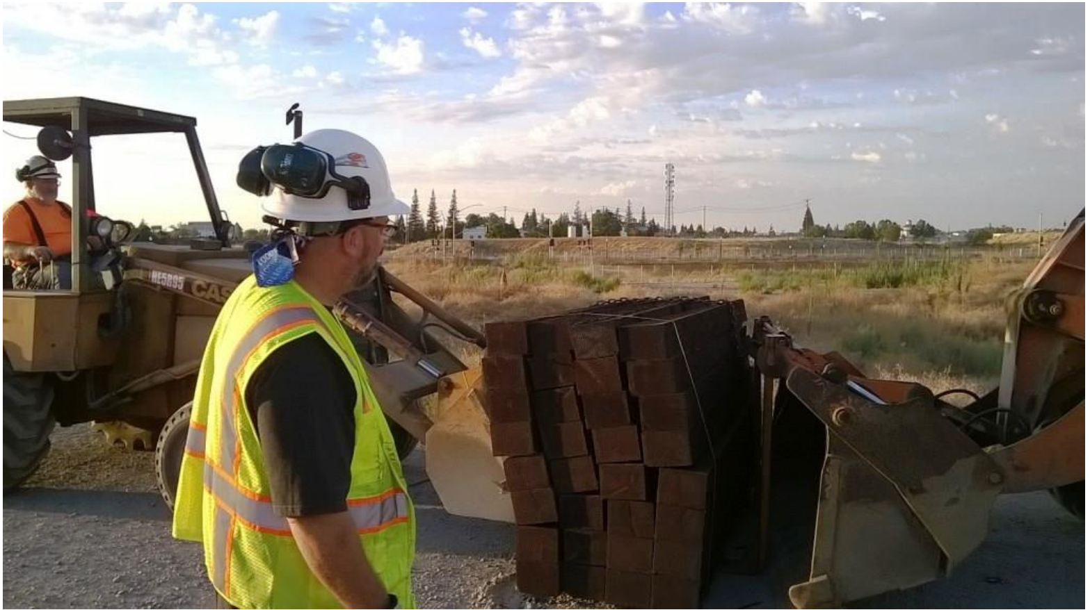
DJ with Frank, on the back-hoe, secure the wobbly bundle of ties to the front-end loader
