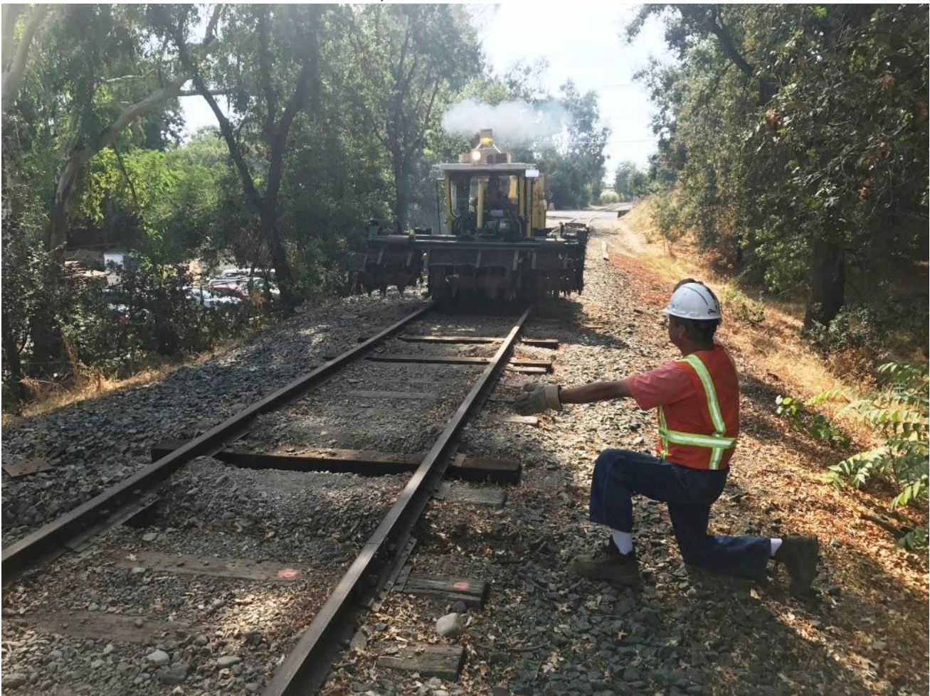
Down near the Zoo, John guides Mike F. to the empty tie-crib to be scarified
