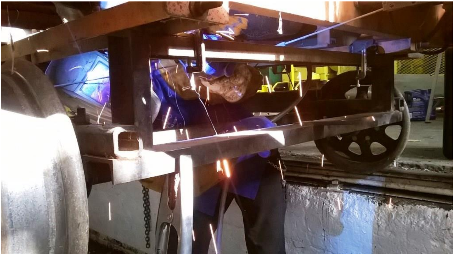
Kyle welds the securing system to the chipper's rail-mounted cart
