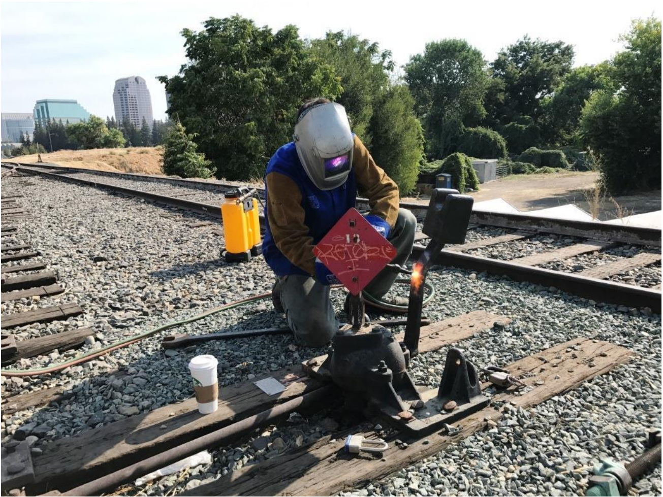
Kyle heats the \frac{3}{4} " thick steel handle to the perfect temperature...
