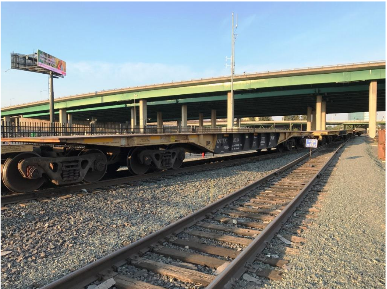
Four flatcars foul the Interchange Track preventing any movement of equipment from the Shops to Old Sacramento
