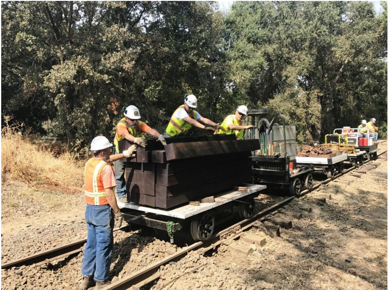
As the tie-cribs were dug out by the scarifier, John, Joe, Kyle, and Taka deploy new ties for insertion
