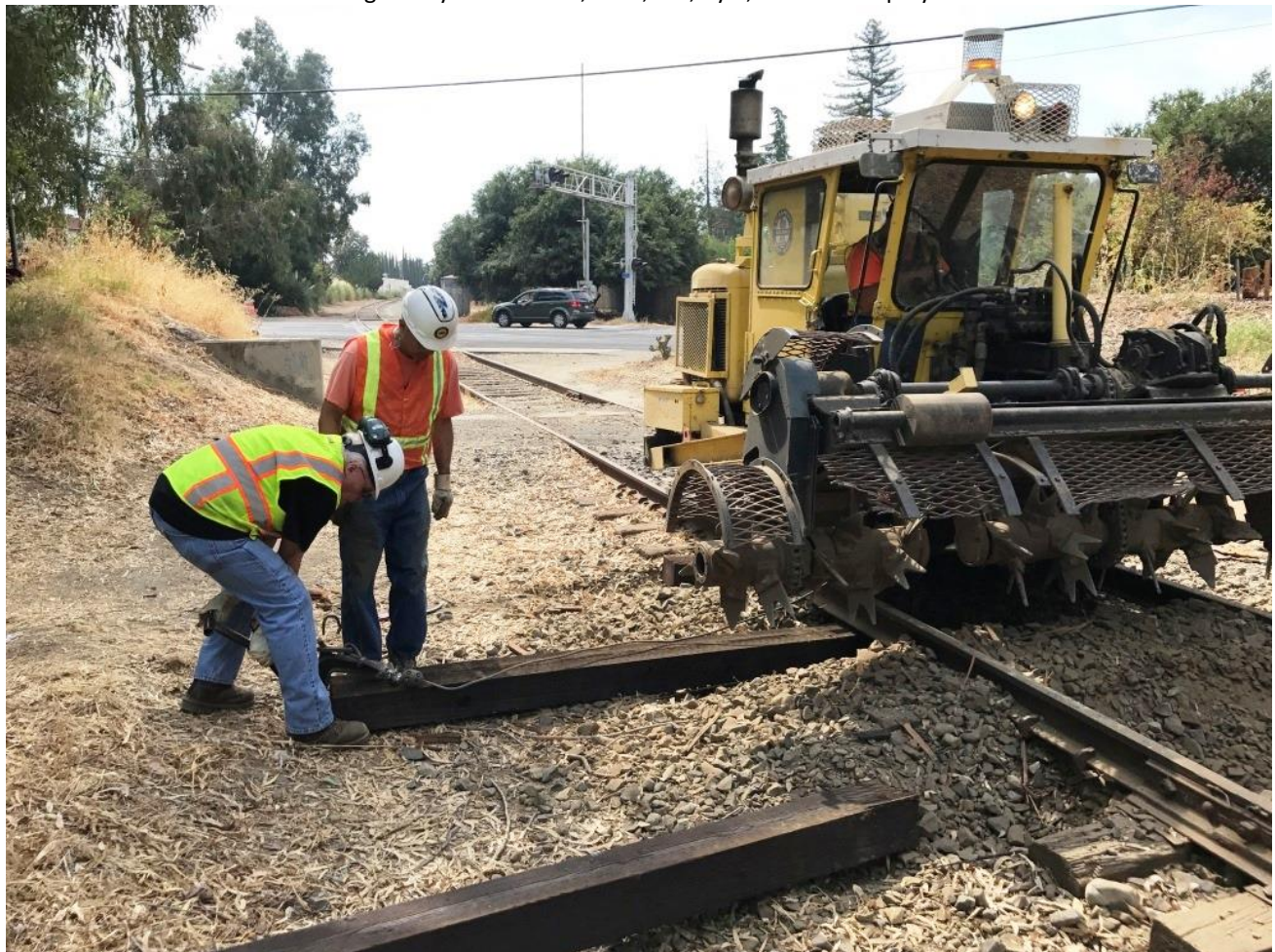
Bill and John hook the inserter function on the scarifier to the new tie
