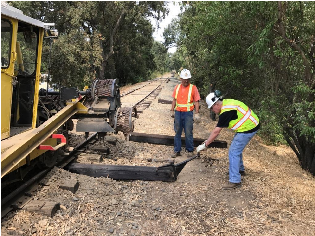
With Bill guiding the tie's path, Mike F. in the scarifier pulls the tie under the rails
