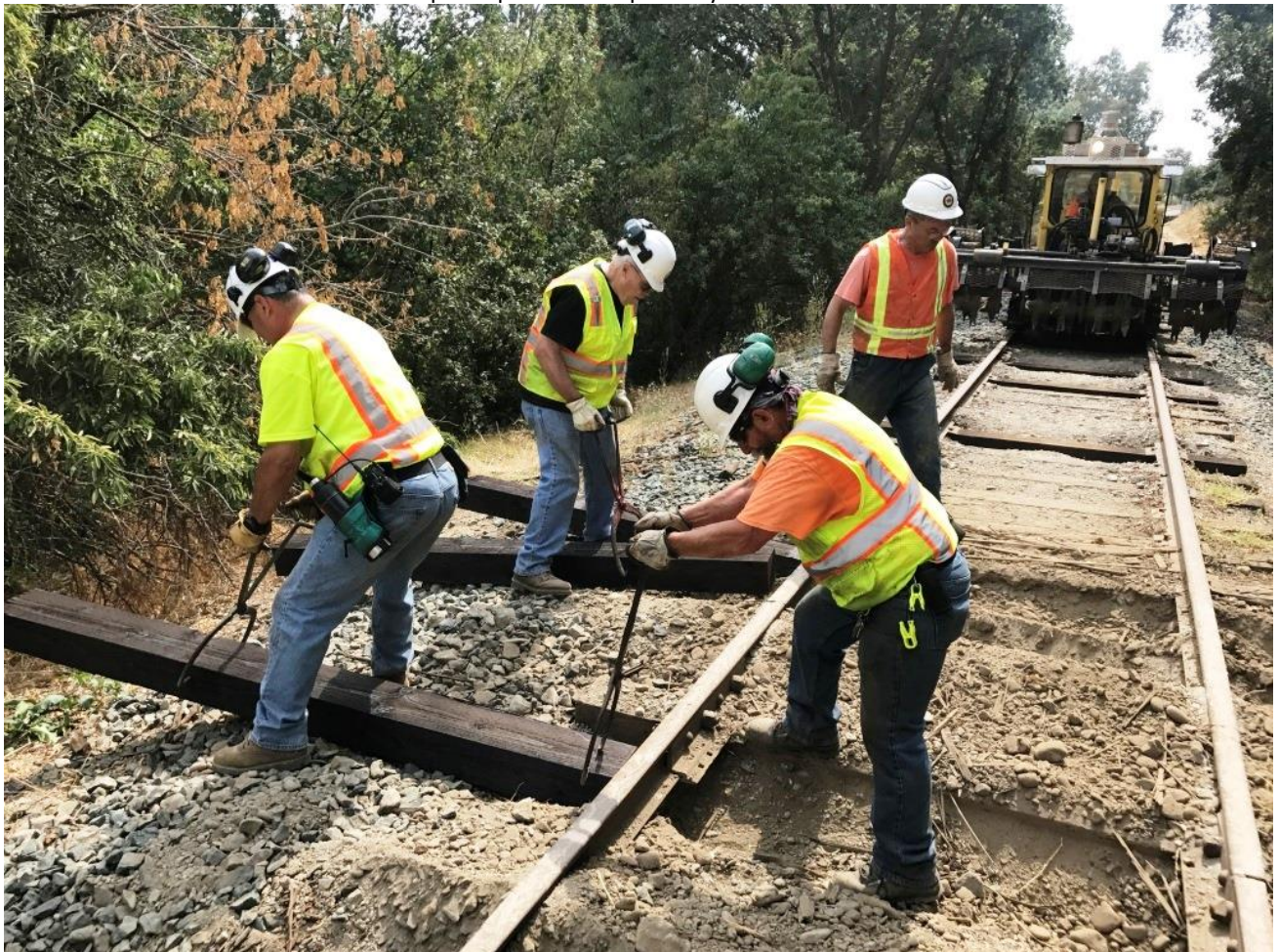
Taka, Joe, Bill, and John get ties lined-up for Mike F. in the scarifier to insert
