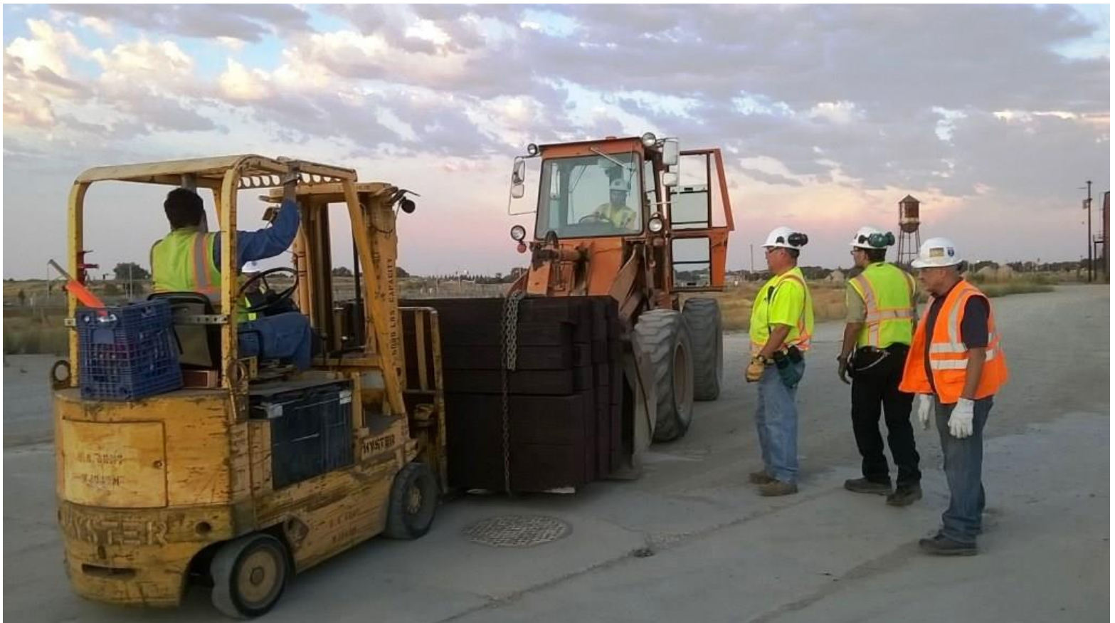
Bundle number two is brought to Joe on the loader by Weston on the forklift which Taka, Kyle, and Dave prepare to chain it down
