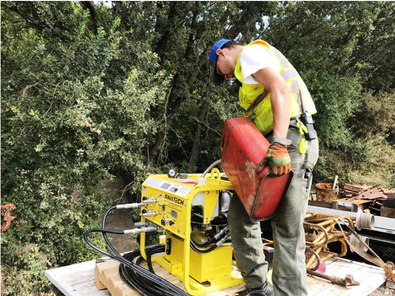
Kyle adds fuel to our super new hydraulic power unit
