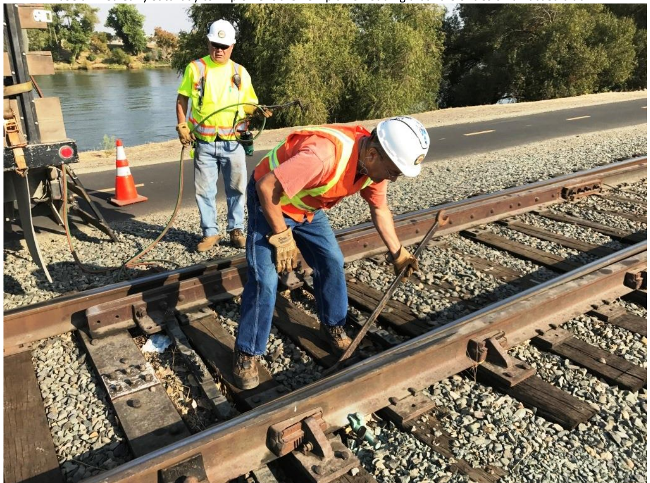
At Switch 13, John removes the point-clamp
