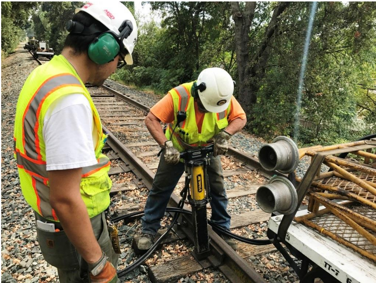
Joe uses the hydraulic spike puller to pull spike on ties slated for removal
