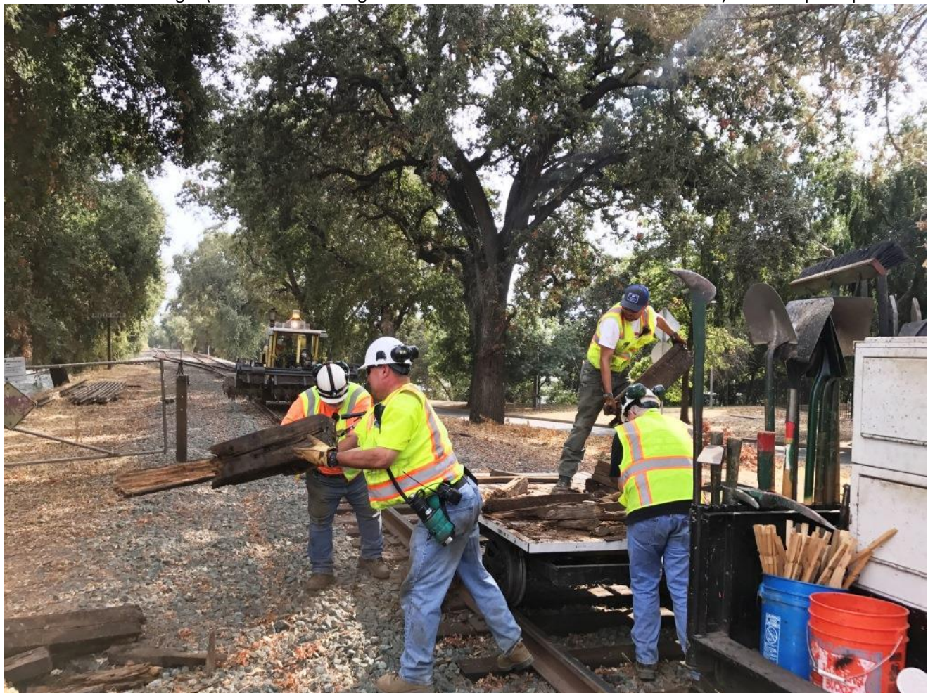
Final task of the day to dispose of tie-sheared tie debris
